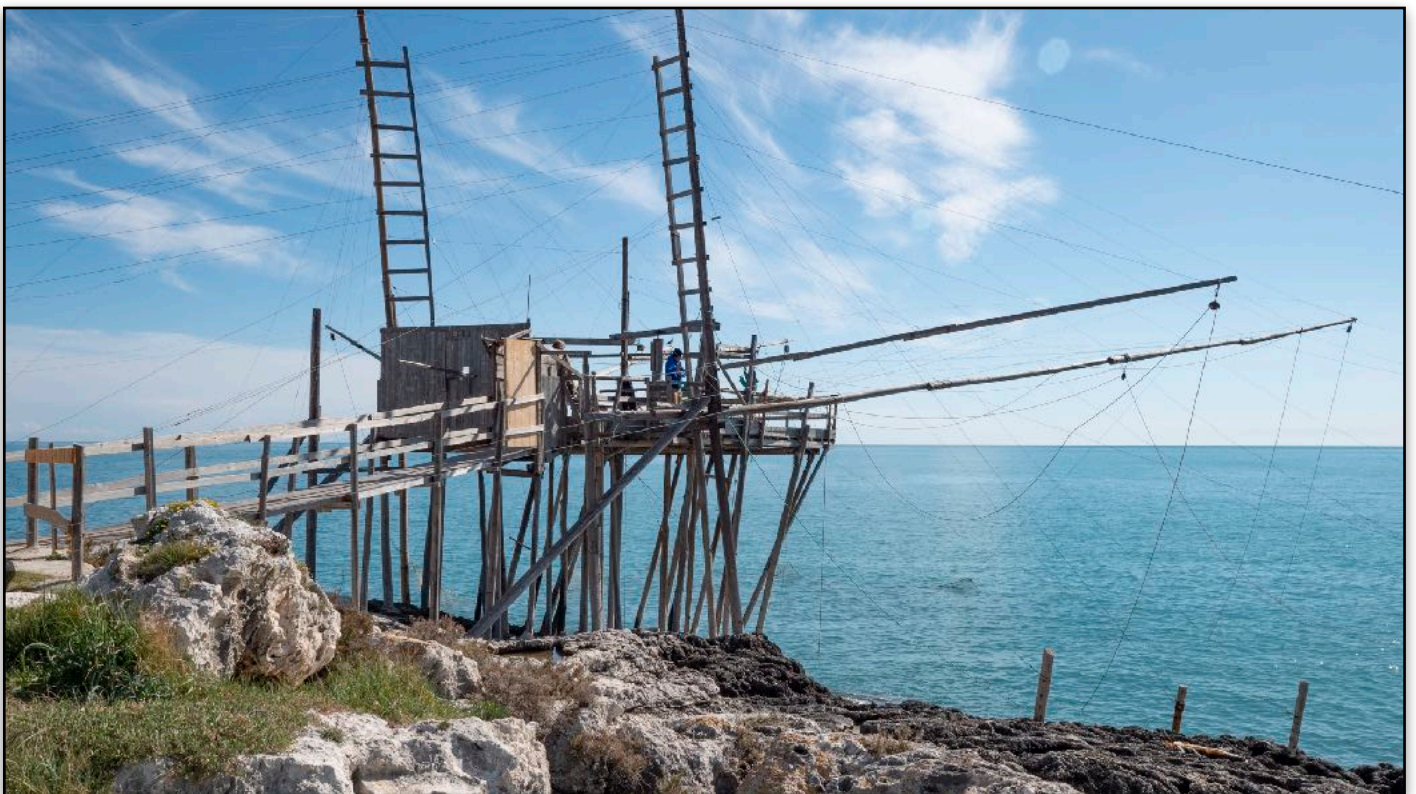
A Trabucco...one of the traditional coastal fish traps with nest lowered and raised by pulleys to catch shoals of fish. This one is about 300 years old but the design dates from Phoenician times..ten times older.
